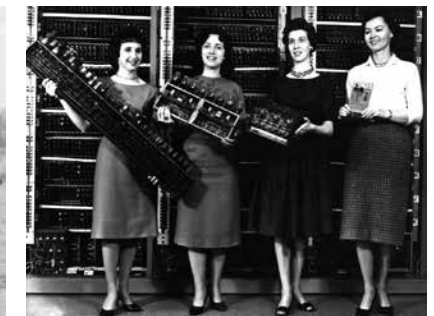
Scientists holding components of the ENIAC Computer they helped to design, c.1948.
