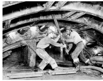
Sandhogs tighten a bolt in a tunnel-lining ring, 1939.
