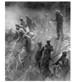
Drillers on the Loudoun Dam, Tennessee Valley Authority, 1942.
