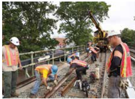
MTA workers repairing track in Queens, 2014.
