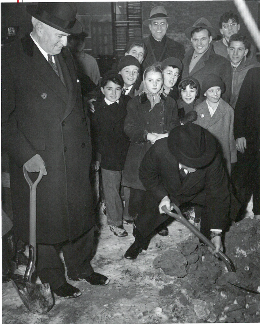
Mayor LaGuardia scoops first earth for $3.9 million Elliott Houses, public housing project in Chelsea, Manhattan, December 20, 1945. New York City Housing Authority Chairman Edmond B. Butler and children from nearby Public School 33 look on.
